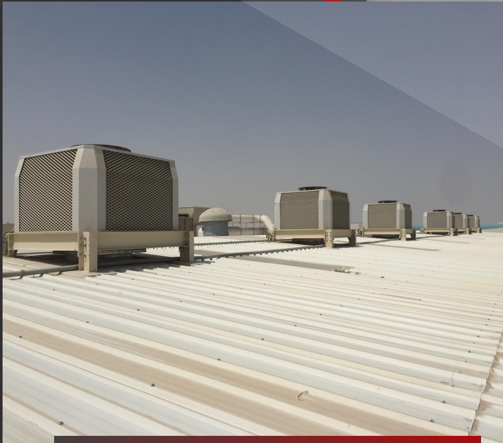
OXYCOM – IBRI OMAN (Ongoing)
