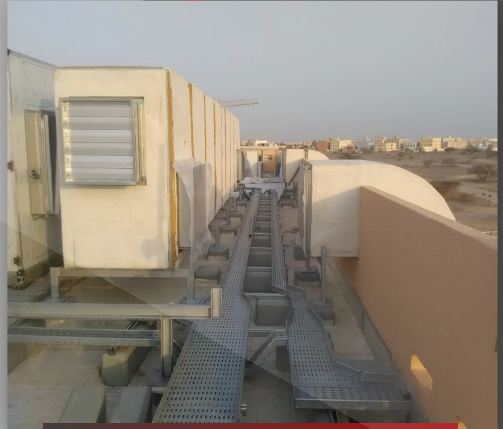
MEP Works – Salalah Jetty Revamp Project 2016
