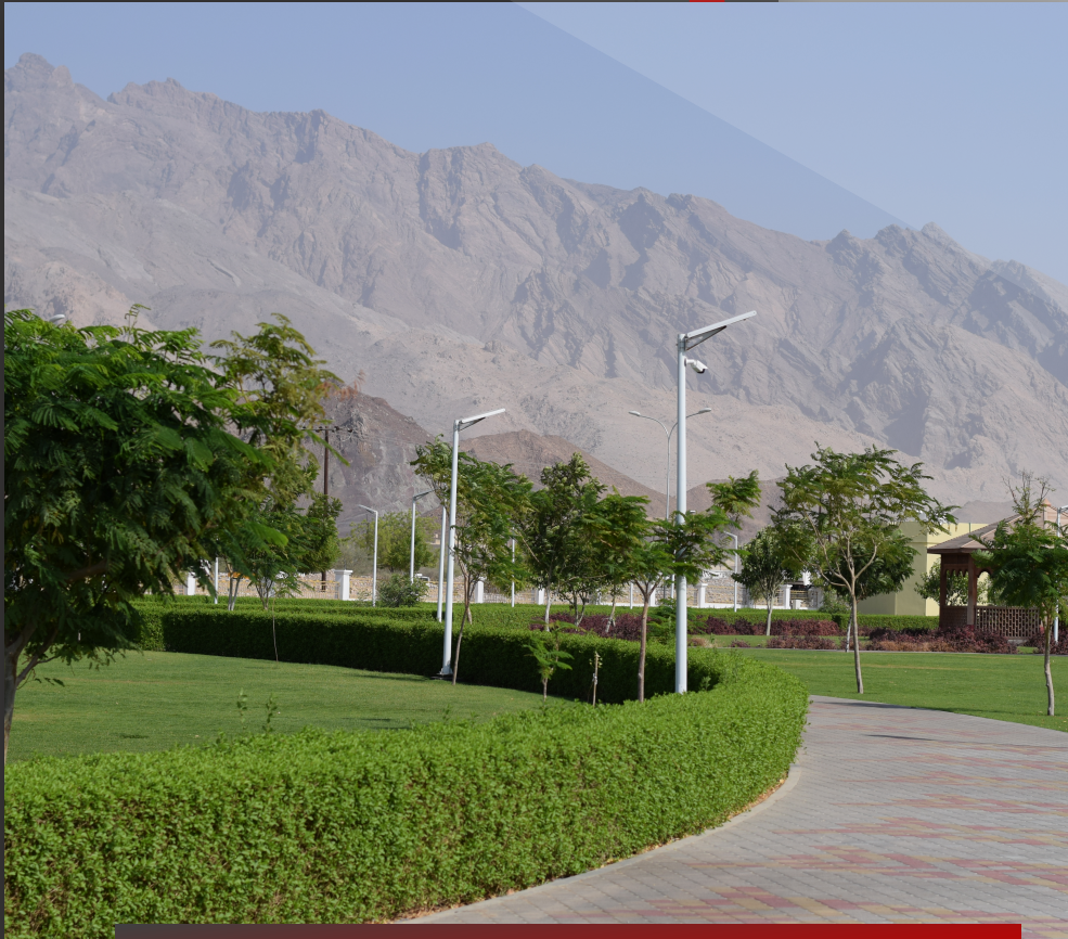
MINISTRY OF REGIONAL MUNICIPAL AND WATER RESOURCES - SOLAR LED IN SAMAIL PARK 2017
