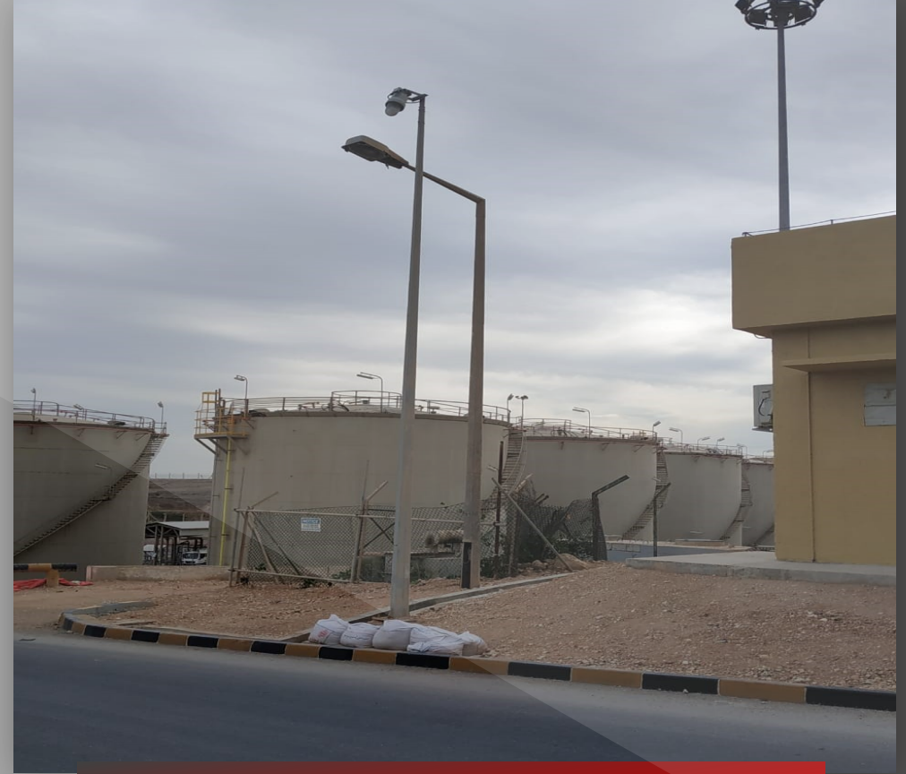
TANK LIGHTING- SALALAH JETTY REVAMP PROJECT 2016
