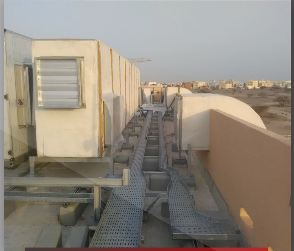
MEP Works – Salah Jetty Revamp Project 2016
