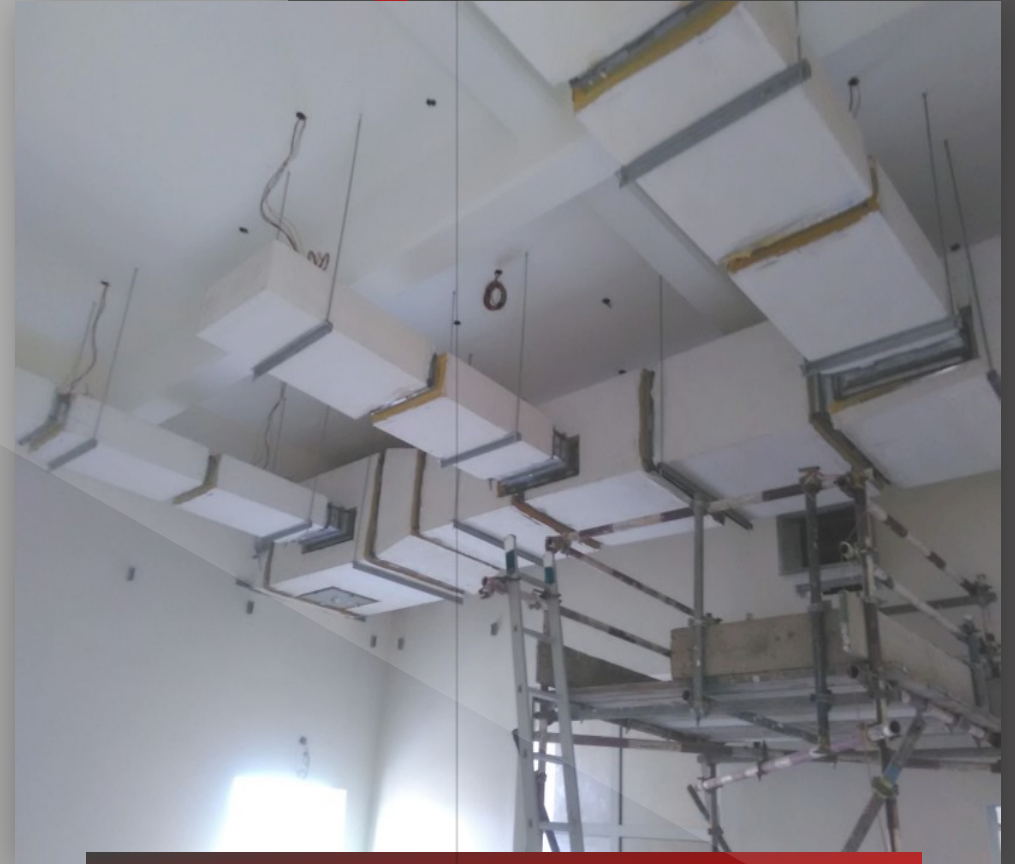
MEP Works – Manah GSS Project 2018
