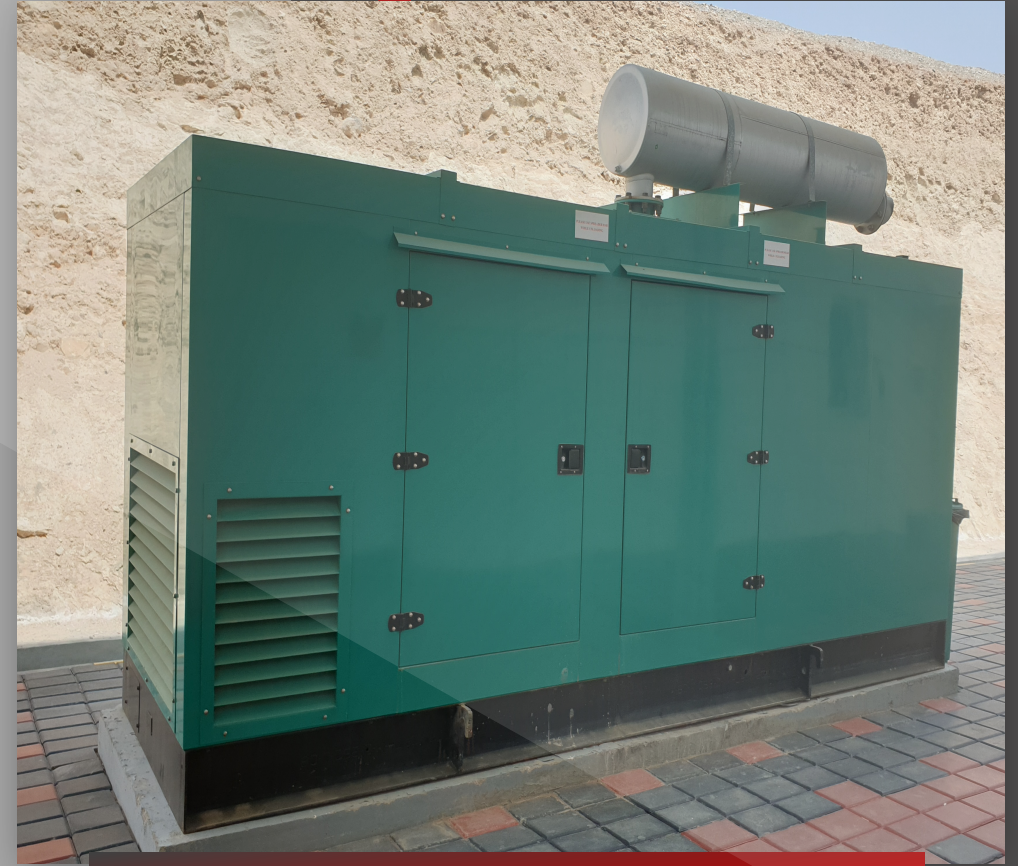
SCHLUMBERGER - DIESEL GENERATORS (250 kVA) 2017
