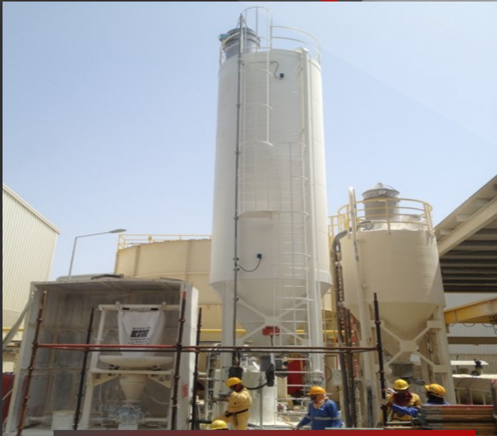
MEP works of Lime Dosing Silos – NOMAC Barka 2017
