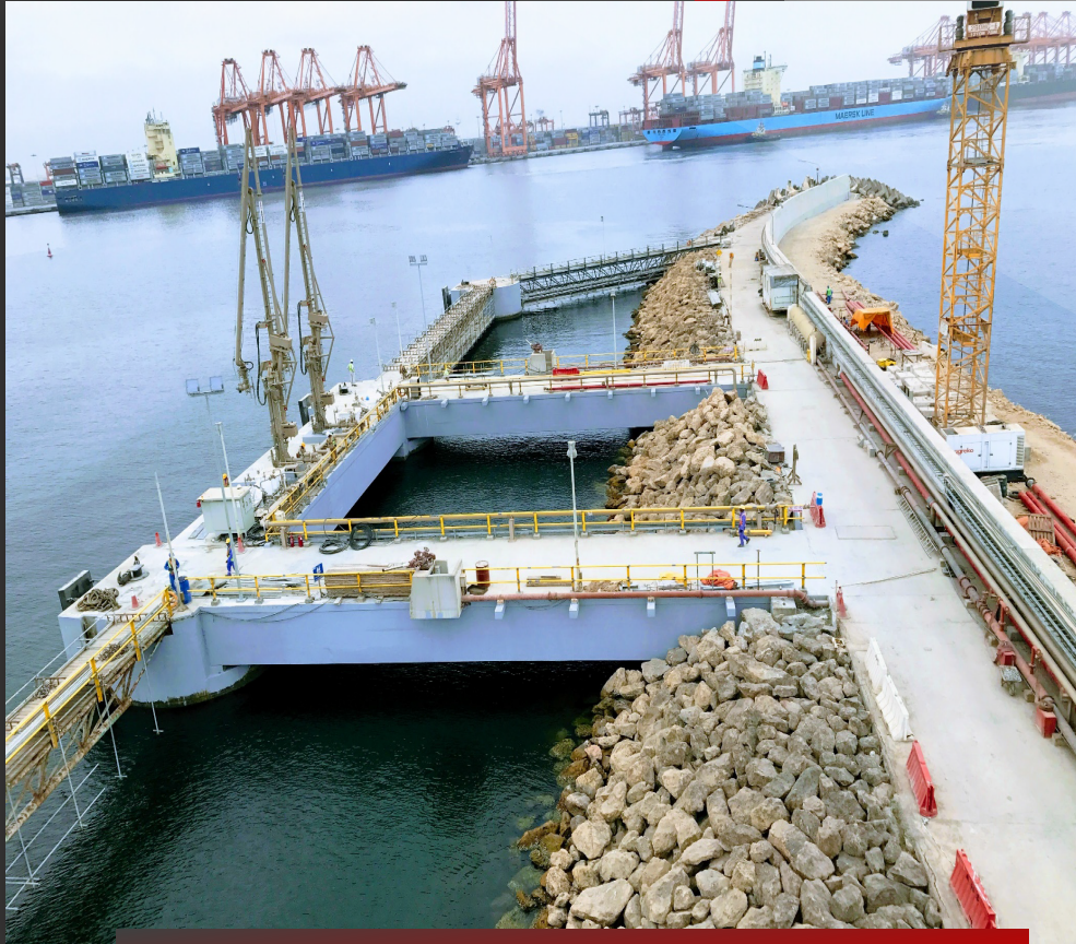
POLE MOUNTED LIGHTS- SALALAH JETTY REVAMP PROJECT 2016
